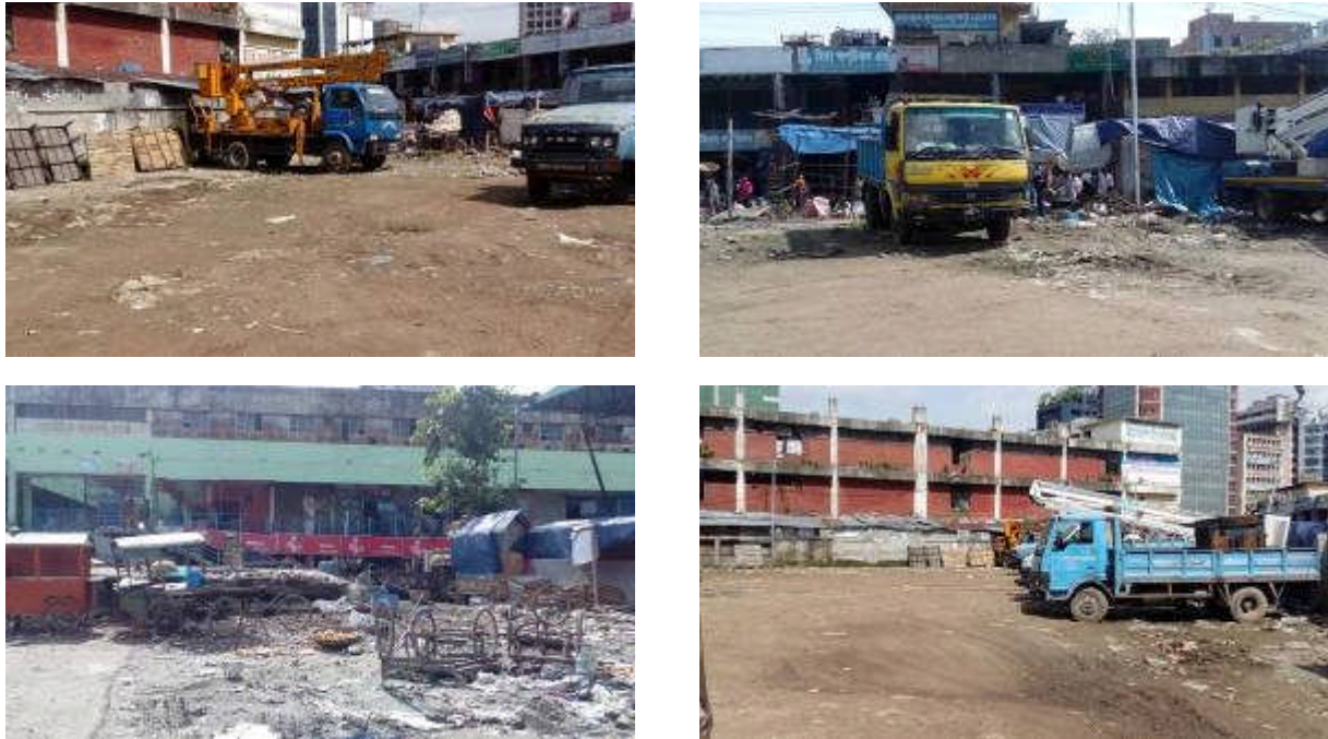
Figure 5: Photograph showing the present condition the sub-project area
