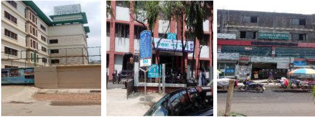
Figure 7: South side major features of the site
